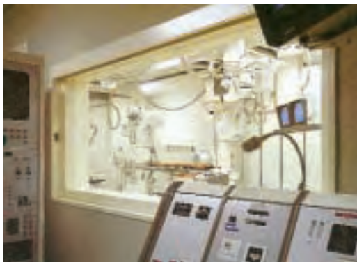
Observation window for angiography room. LX lead glass is manufactured by Nippon Electric Glass Co. Ltd. Japan
