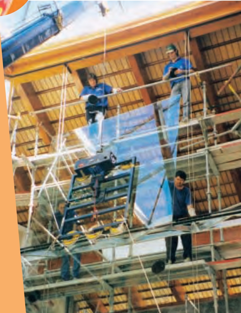
Figure 11.2a: Example of Dry Glazing
