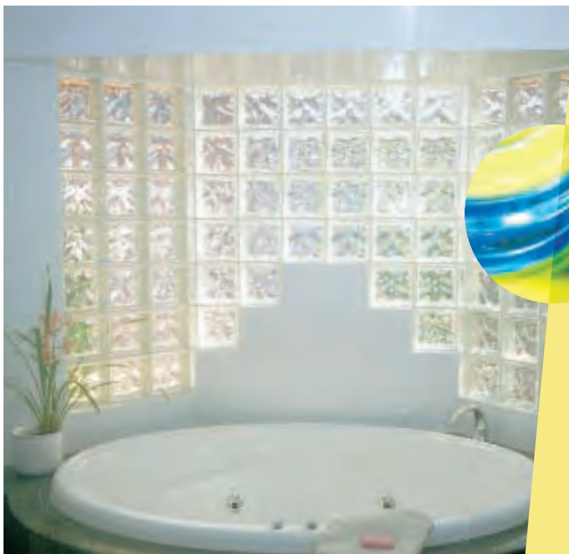
Glass blocks used in bathroom application
