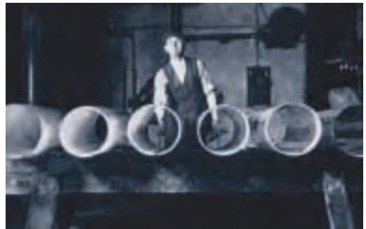
The old cylinder process
